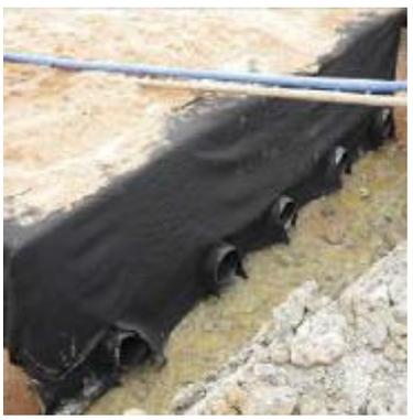
Five low flow channels connecting 150mm inlets to 300m outlets
