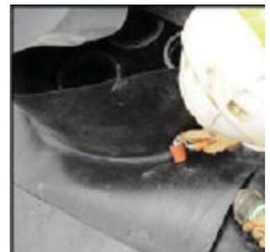
Preformed tuflex cloaks are heat welded to inspection chamber openings
