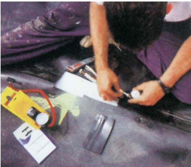
Pressure testing of welded joints (part of standard CQA procedures)
